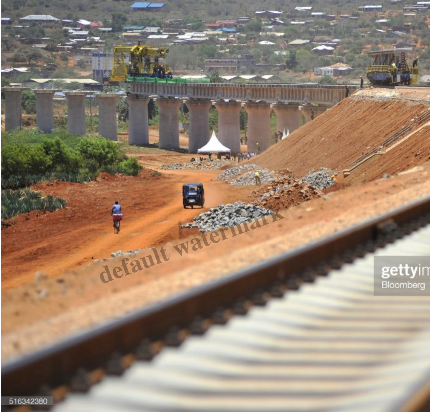
A wagon carries a pre-formed bridge section towards the raised supports of a new superbridge which will form part of the new Mombasa-Nairobi Standard Gauge Railway (SGR) line, in Voi, Kenya, on Wednesday, March 16, 2016. By providing an alternative to roads, the 1,100-kilometer (684-mile) Chinese-financed railway will slash the time and cost of transporting people and goods between East Africa's landlocked nations. Photographer: Riccardo Gangale/Bloomberg via Getty Images
